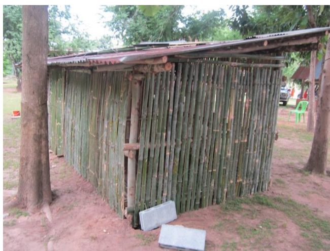
Figure 3 The roof sloping backwards housing, roof with zinc, bamboo for construction and ground for floor were the most favored for farmers in this study
